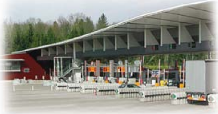
Road traffic management
