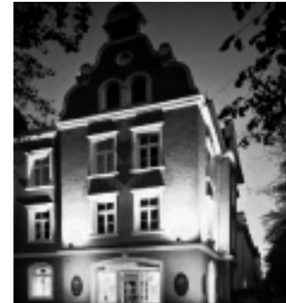
Architectural lighting with EFFECTlight
